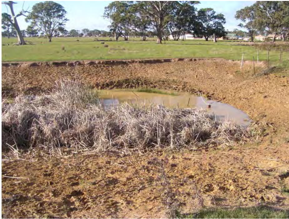
Photo 5 The existing dam in the middle of the depression will be integrated with the proposed wetland system. The exposed soil profiles and muddy water reveal the dispersive nature of the subsoils. All water bodies will need to be fully covered by suitable depth of topsoil to mitigate subsoil dispersion into the water column.
