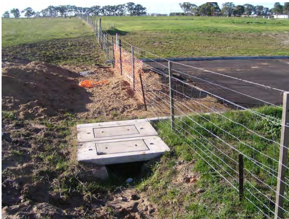
Photo 2 The existing Ashley Street construction and inlet to 1050 mm pipe drain at east boundary of site, looking northwards towards the nursery and Bairnsdale-Paynesville Road.
