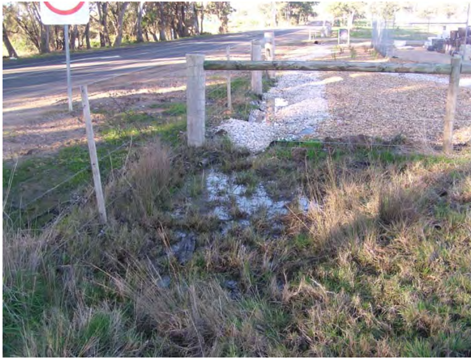
Photo 1 The northeast corner of the site showing swampy ground conditions on frontage to Bairnsdale-Paynesville Road and the nursery caused by failure of earlier developments to provide for natural surface drainage at this location. It is proposed to redirect all pipe drainage from the new development southwards to resolve this problem.
