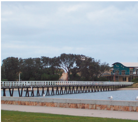
Pedestrian bridge across to ocean beach
