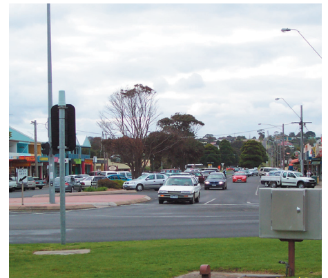
Improve open space opposite Myer Street
