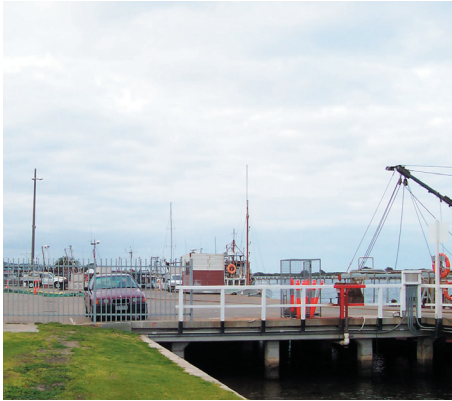
Gippsland Ports Yard
