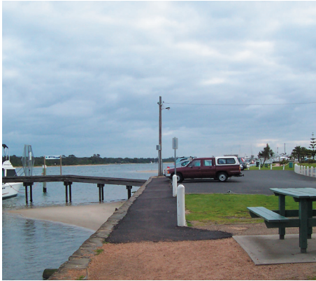
Inconsistent footpath treatment along foreshore
