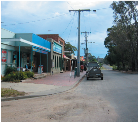
Streetscape improvements required
