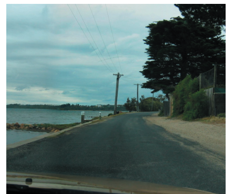
Improve pedestrian access on western side of Shaving Point
