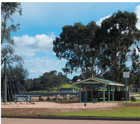
Upgraded foreshore with Playground & Picnic Shelter
