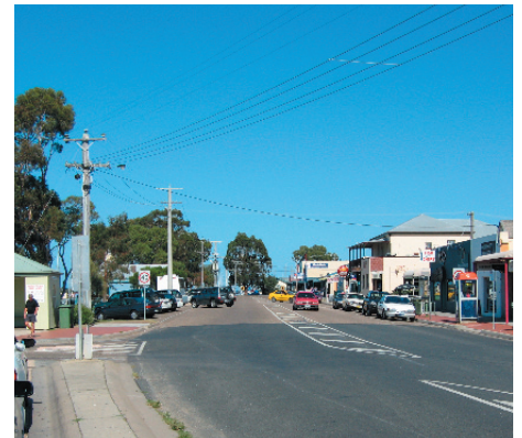
Remove overhead powerlines along Esplanade
