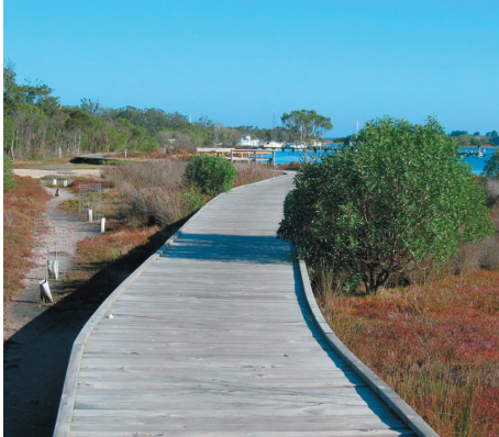
Boardwalk on McMillan Strait foreshore
