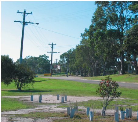
Overhead powerlines on Western Boulevard
