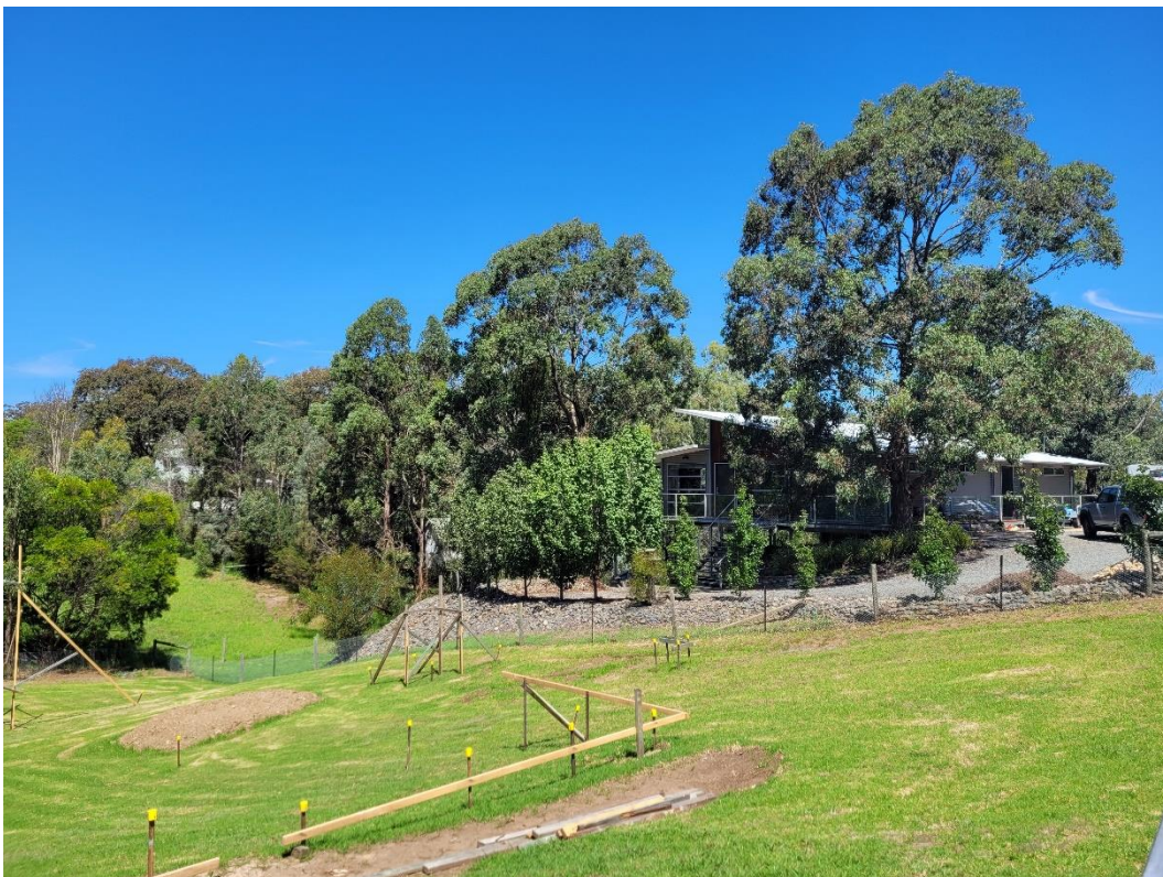
Photograph 5 – Subject site at 35 Muir Place facing south.
